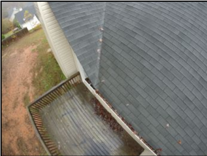
Clean gutters: Significant amounts of debris evident.
