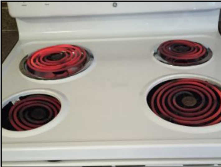
Functioned properly, but front two eyes missing drip pans.
