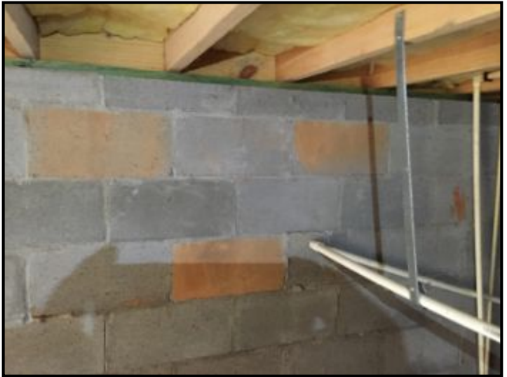
PVC drain pipe leaving heater has swag where water cannot effective drain - recommend fixing to where there is a continual slope downward to this pipe for proper drainage.
