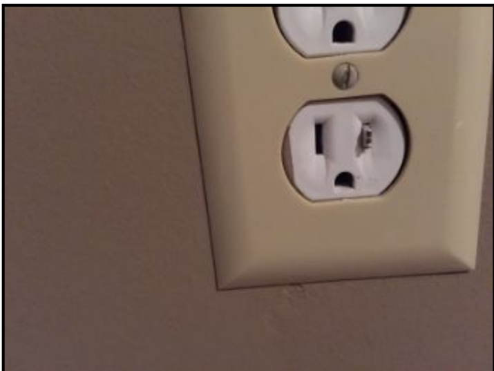
Prong broken off inside outlet - should be replaced.
