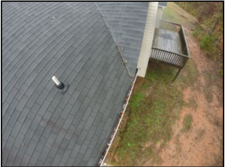
Clean gutters: Significant amounts of debris evident.
