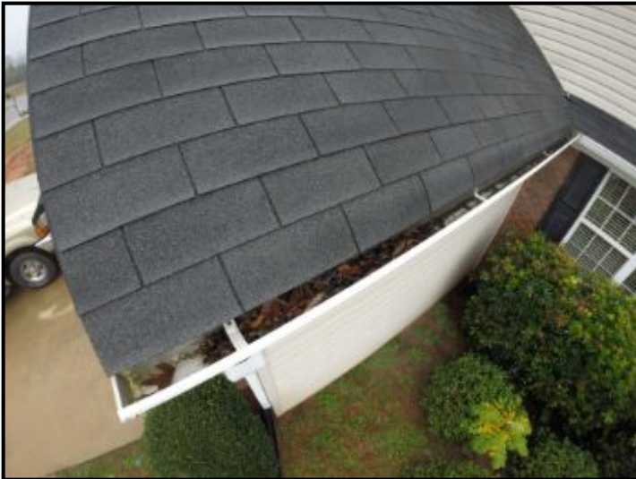
Clean gutters: Significant amounts of debris evident.
