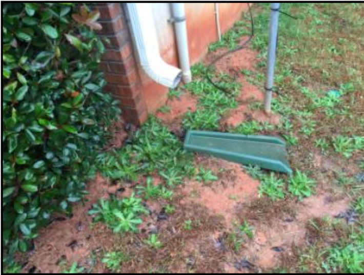
Downspout should be installed closer to the ground to keep water from impacting ground and causing holes if splash guard is moved.
