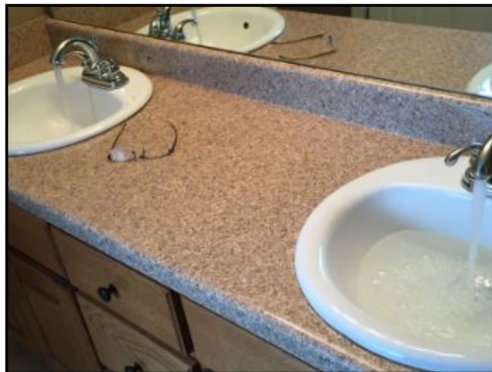
Slow drain at right sink in master bedroom. Recommend clearing.
