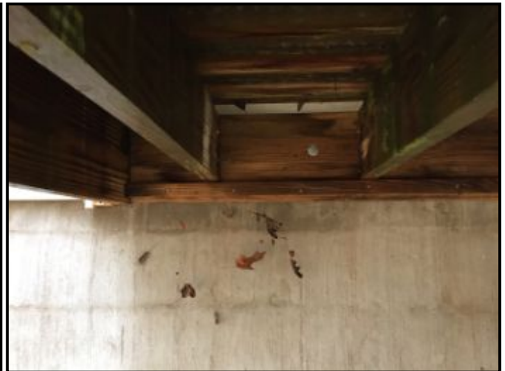
Porch deck bolted into side of house.
