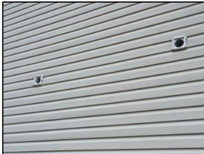
Two vent covers missing on outside of siding.
