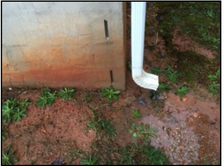
Missing splash plate.
